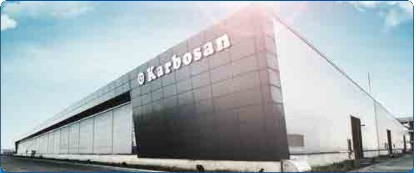
Karbosan Velikoy Plant
